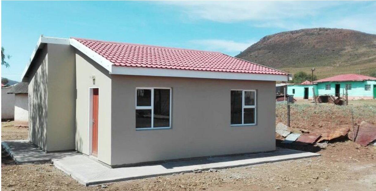
ABOVE: A “Malibongwe” designed house, one of the sixty completed houses.
