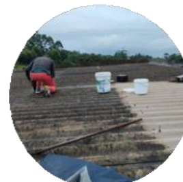
Nethezeka cleaning services cleaning the roof of one of their customers.
